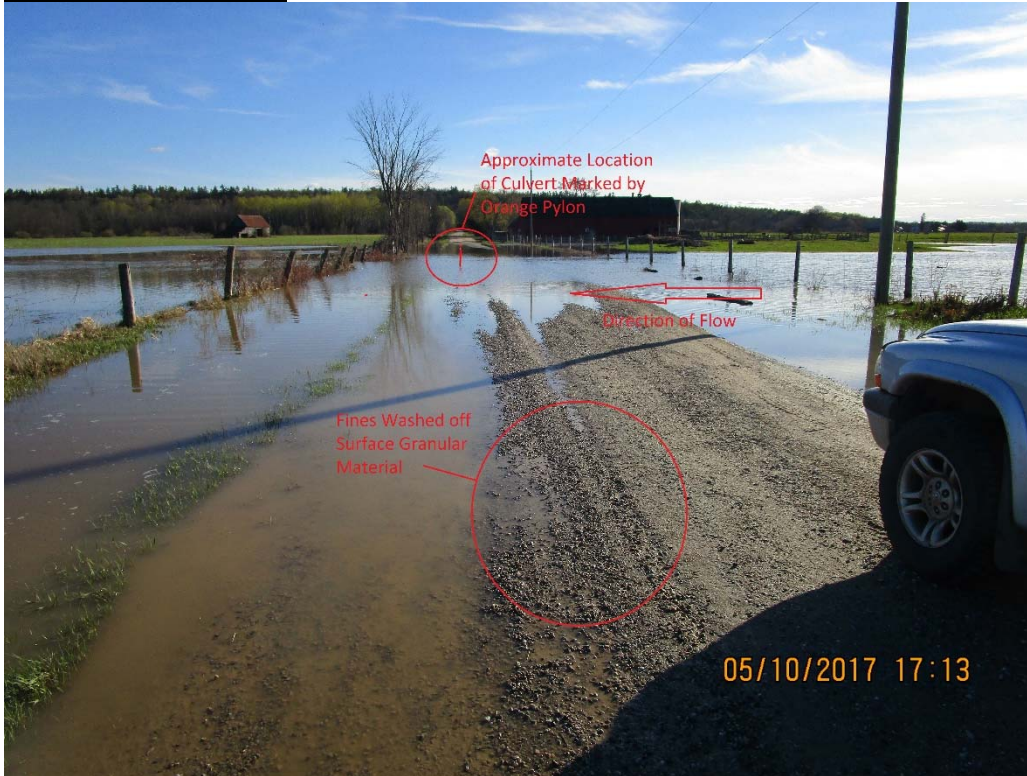
Figure 1: Photo of flooded culvert section facing south towards River Road depicting the extent of the flooding and location of the culvert.
