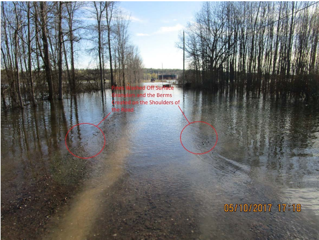
Figure 6: Photo taken facing south towards River Road depicting the berms created on the shoulders by the coarse granular material.
