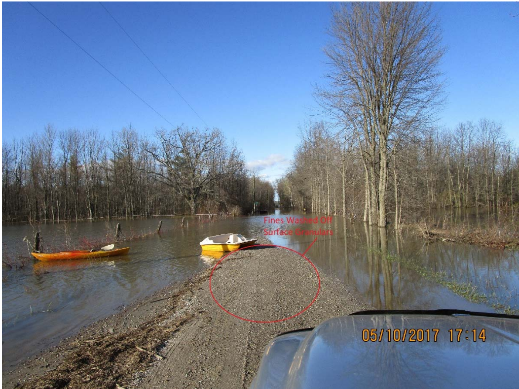
Figure 5: Photo taken facing north towards the Ottawa River of flooded dead end section showing extent of flooding and the granular material washed off the road.
