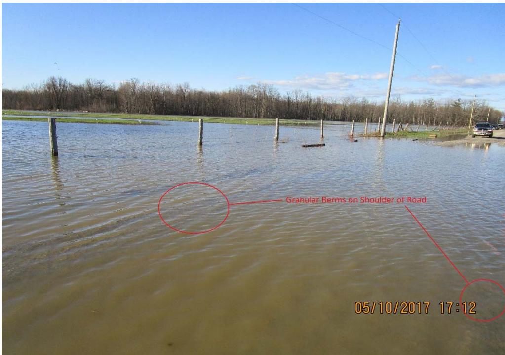
Figure 3: Photo depicting the berms created on the shoulders of the road.
