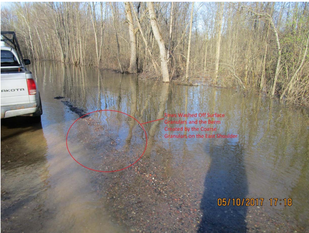
Figure 7: Photo of the east shoulder of the road depicting the fines washed out of the surface granular material.
